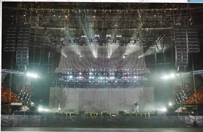
ABOVE: BOTH ELEMENT LABS STEALTH SCREENS VISIBLE AND BEING POSITIONED VIA VARIO LIFT SYSTEM.
